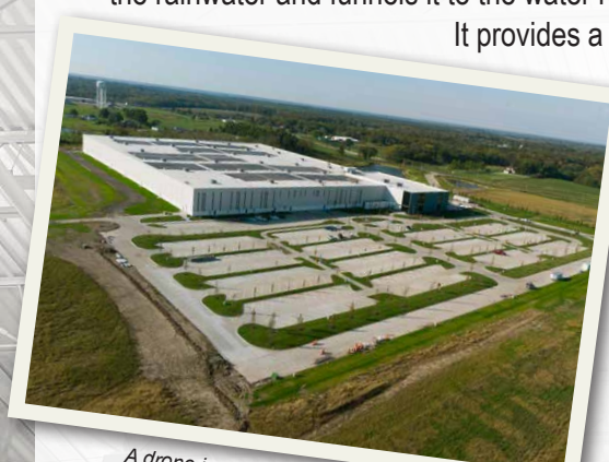
A drone image from the north, showing Employee parking lot north of the building and expansion area to the east. Landscaping mostly in place. Image by Jarrod Schwartz 10-26-21
