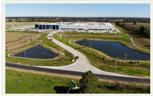
A drone image from the west, showing the trucker’s entrance, dock doors and water retention pools. The blue corner on the left is offices and break room. Air conditioners and solar panels are visible on the roof. Some of the landscaping is visible. Photo by Jarrod Schwartz 10-26-21.
